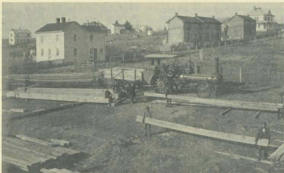
A scene in Woodstock about 1906 showing the largest steam engine that ever operated in Shenandoah County. The engine supplied the power for sawing the lumber and heavy timbers on the Spiker tract near Saumsville, and then hauled it (as shown here, with its tender of firewood) to the loading yard at the railroad tracks, just out of sight at lower left. High Street runs up the hill (west) in front of the houses. Of the seven men in the picture, four are here identified: Henry G. Banning, owner of the operation and the equipment, is holding his horse, Tony; 2d left from him (sitting) is J. D. Grabill; the man in front of the large tractor wheel is Charles Mowery, engineer; and Harvey McInturff (farthest right). (Photo courtesy Fred Painter)
