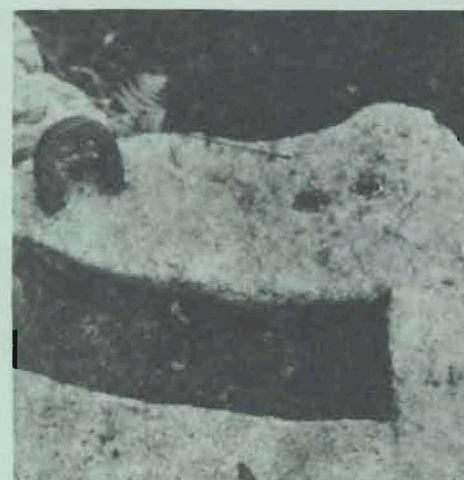
Tie iron set into the stone of one of the locks. The elongated hole was related to the gate mechanism. (Photo by Tom Hahn)
