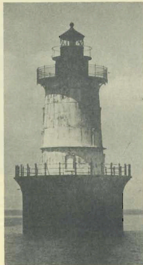
Hooper Island Light, located south of Cambridge, Maryland, and approximately opposite the mouth of the Patuxent River, began operating in June 1902 and has been in continuous operation ever since. It now operates automatically, with batteries and generators as its source of power. The base is 33 feet in diameter, and stands in 20 feet of water. (Photo courtesy Robert de Gast)
