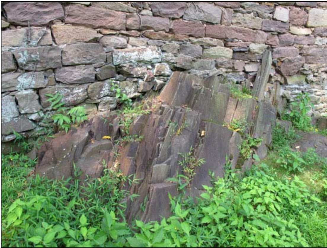
Figure #80: Vertical sheets of diabase bedrock underlying Buckland Mill foundation.
